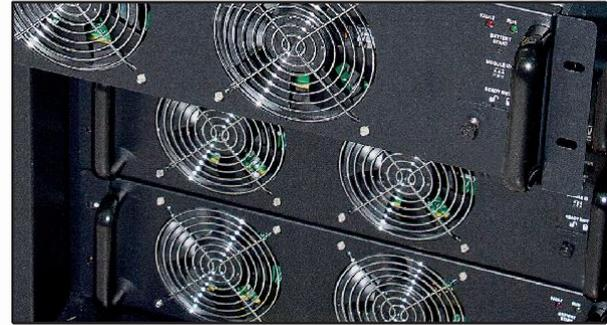
The new modular UPS series JOVYFLEX offers an extremely flexible solution for power supplies from 20 kVA up to 210 kVA. The UPS systems are based on 20 or 30 kVA power modules as well as a static switch 120/180 or 210 kVA / kW. The UPS modules impress with efficient power control, dynamic transitions without switchover times and a high efficiency of 95%. The modular UPS systems JOVYFLEX are the first choice especially for use in data centers.
